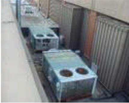
Confined installation traps the hot air then recycles it to try and cool again. This alone and take into consideration the Urban Heat Island effect, these units are in need of an Evaporative Fluid Cooling Tower. We make comfort affordable and energy efficient.
